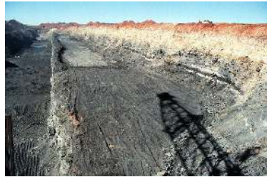
Overburden removal, bench, road & ramp levelling
