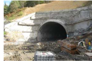
Tunnel driving, roof, face & rib scaling, floor levelling
