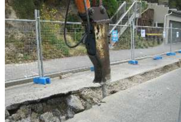
Trenching, pit building, ground excavation
