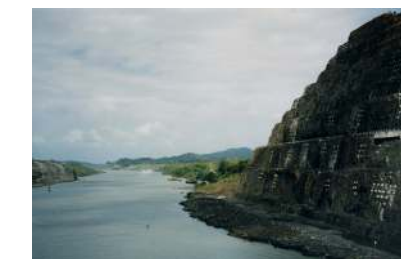
Canal deepening & extension
