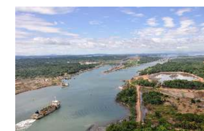
Dock deepening & extension
