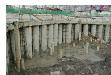
Foundation pile driving
