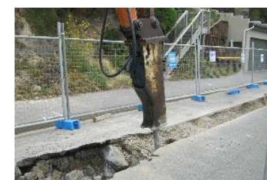
Trenching, pit building, ground excavation
