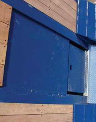
Bucket Plate on Rear Main Deck
