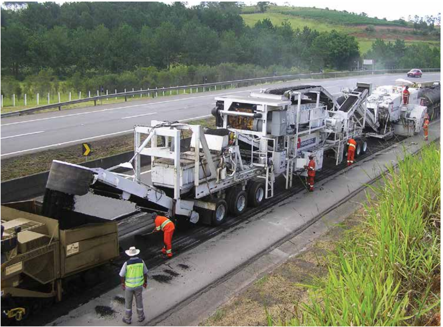
Conveyor discharges directly into the paver
